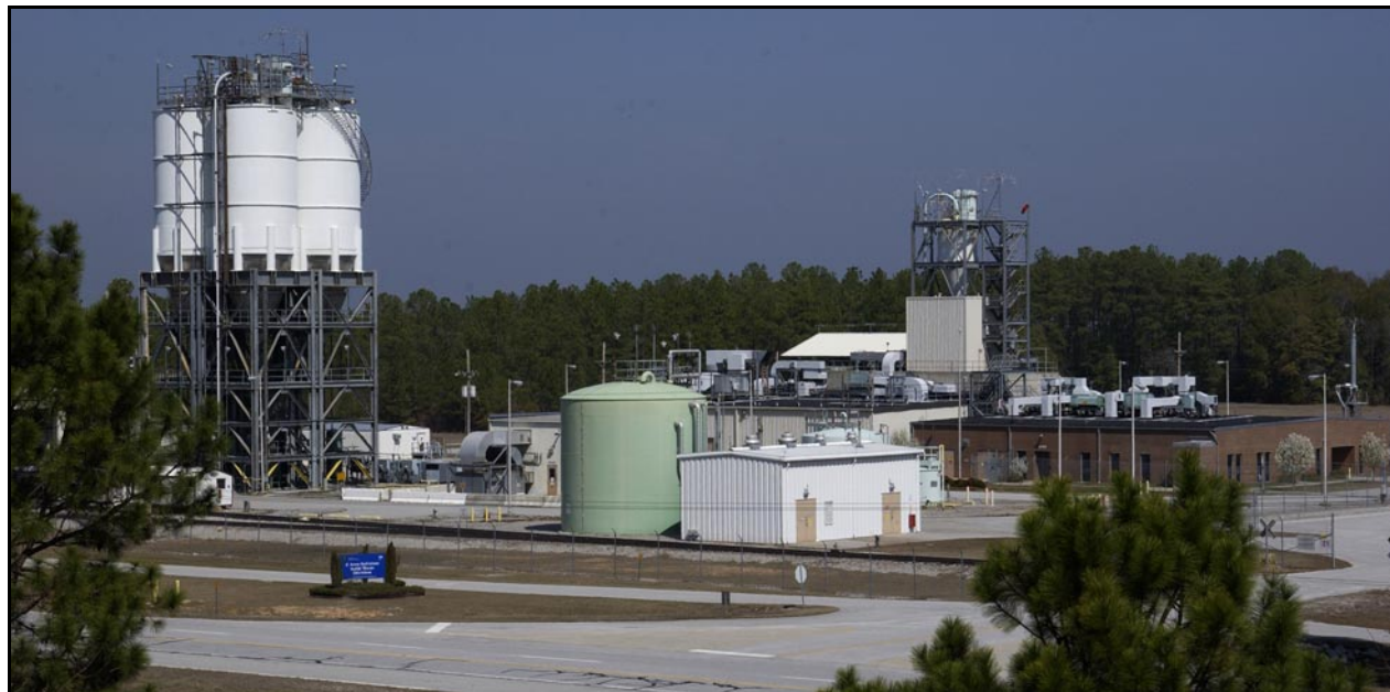
View of Saltstone Facility
