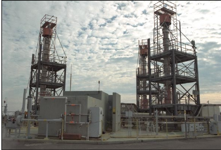
Typical Waste Removal equipment includes three to four 45-foot long slurry pumps and one transfer pump or jet. Note the substantial structural steel required to support the loads in the picture above. At right is the typical installation of a transfer pump (Tank 8) requiring difficult, high-risk entries into High Level Waste Tanks.
