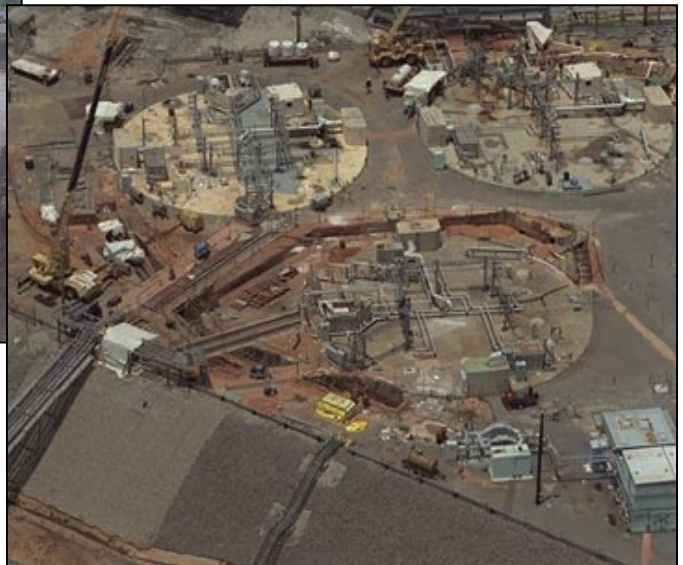
Overhead View of H Tank Farm showing the tops of three tanks. Each tank is approximately 90 feet across and can contain over one million gallons of waste.
