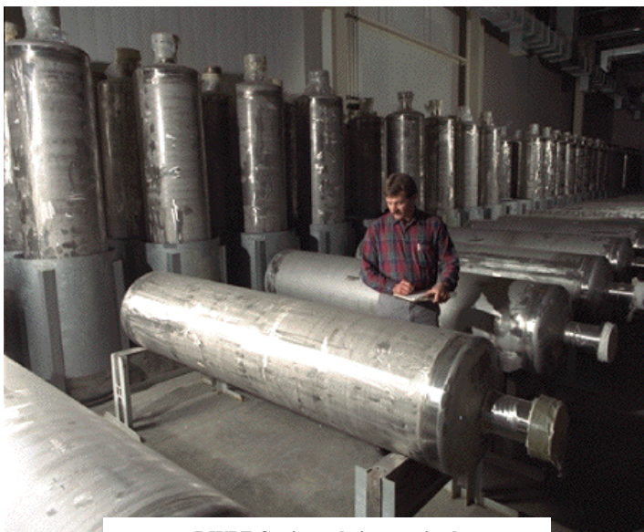
DWPF Canisters being received (prior to being filled with Radioactive Glass)
