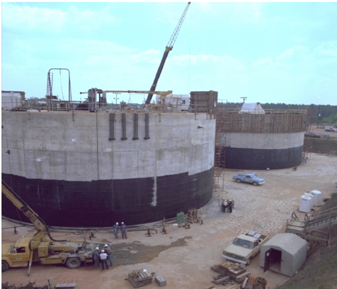
Tanks under construction. Note tank size relative to construction workers. Later, dirt is backfilled around the tanks to provide shielding.
