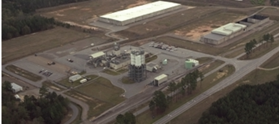
View of Saltstone Facility: Processing Facility in foreground, two vaults in rear.
