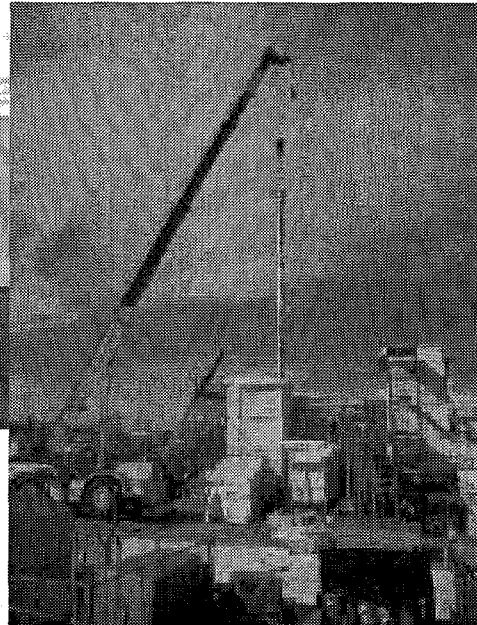
Typical Waste Removal equipment includes 3 to 4 45-foot long slurry pumps and one transfer pump. Note the substantial structural steel required to support the loads in the picture above. At right is the typical installation of a transfer pump, requiring difficult, high-risk entries into High Level Waste Tanks.
