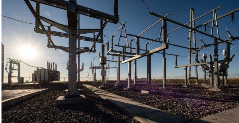
The Flatirons Campus substation at NREL is part of the Power Generation Upgrade Project, which is changing the source of utility power at the Flatirons Campus from the distribution network that feeds businesses and houses to the transmission network that ties all the power plants and substations together. Photo by Dennis Schroeder, NREL
