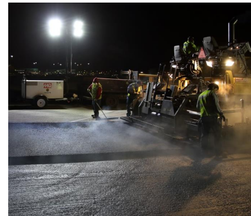
Runway repair operations 7-28-14
