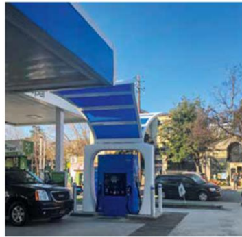
Refueling station in Oakland (California)
