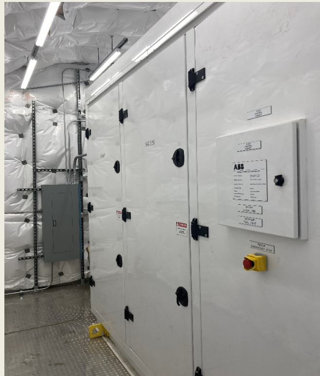
Hughes 250kw/335kWh ABB Emesh unit inside Quonset Hut
