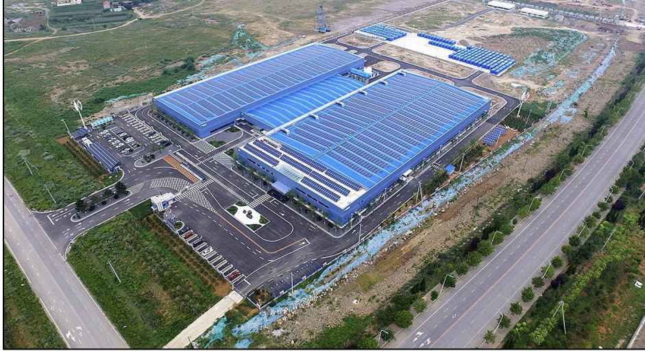
Figure 40. Largest vanadium redox flow battery facility (under construction)
