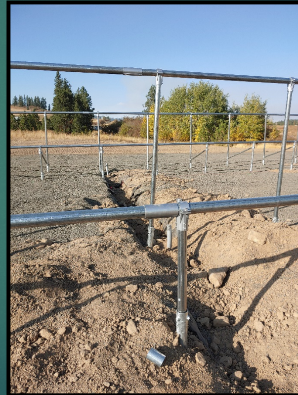
Installing the racking
