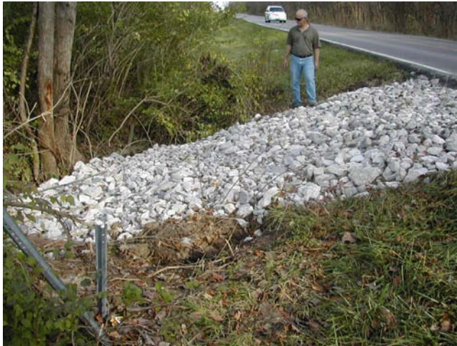
Photo 10. Gravel repair to Highway D Culverts.
