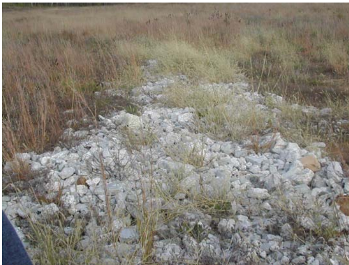
Photo 22. Erosion control repairs.
