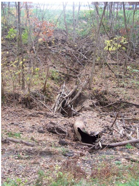
Photo 12. Highway 94 culvert inlet in the Southeast Drainage.
