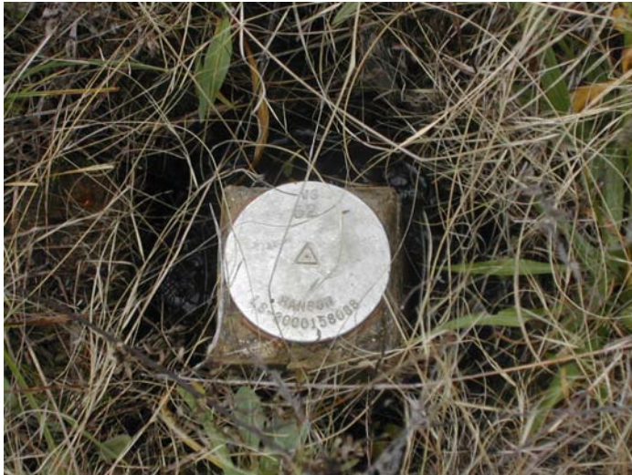
Photo 4. Groundwater restriction boundary monument WS-52. Has been dug around sides.
