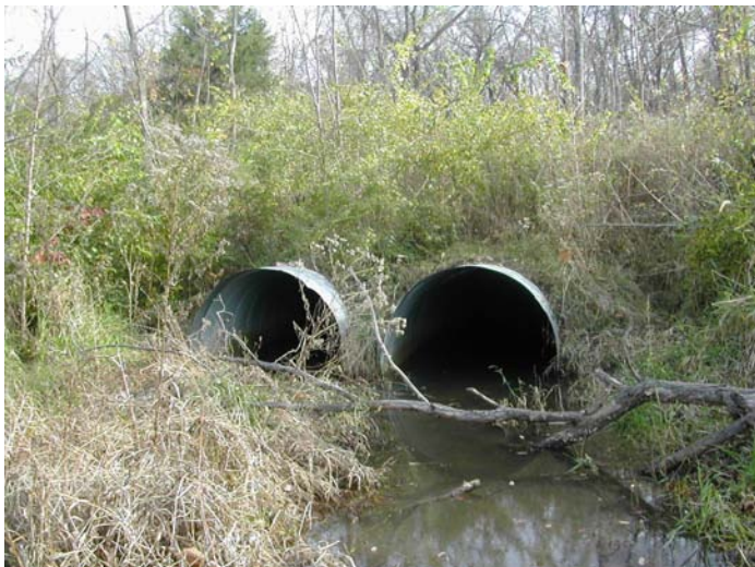
Photo 9. Outlet end of Highway D Culverts.
