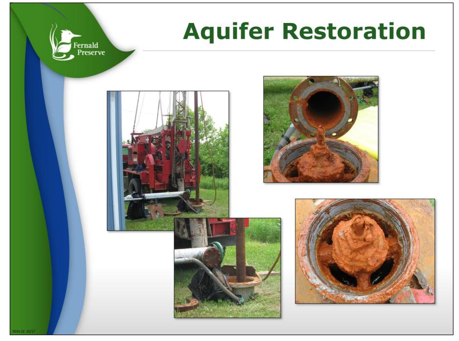
Four wells were rehabilitated in 2016 to address iron plugging. Iron plugging decreases the pumping efficiency of the well.
