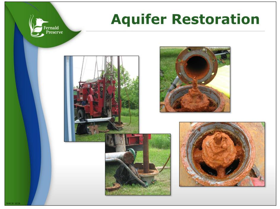
Five wells were rehabilitated in 2017 to address iron plugging. Iron plugging decreases the pumping efficiency of the well.
