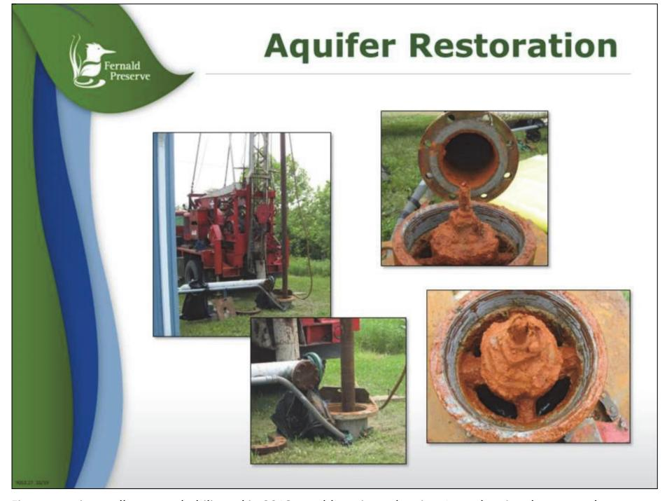
Five extraction wells were rehabilitated in 2018 to address iron plugging. Iron plugging decreases the pumping efficiency of the well.
