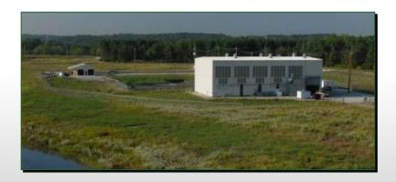
The aquifer cleanup, which involves pumping and treating water from the aquifer, is progressing as planned. Groundwater modeling projects that aquifer cleanup will be completed in 2026. Since 1993, over 9.85 billion gallons of groundwater have been treated.
