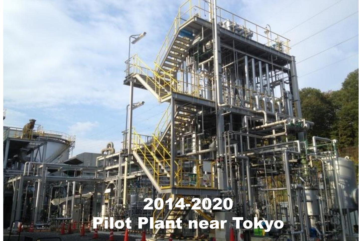
**World-first demonstration of continuous direct ethanol production from MSW-derived syngas**
