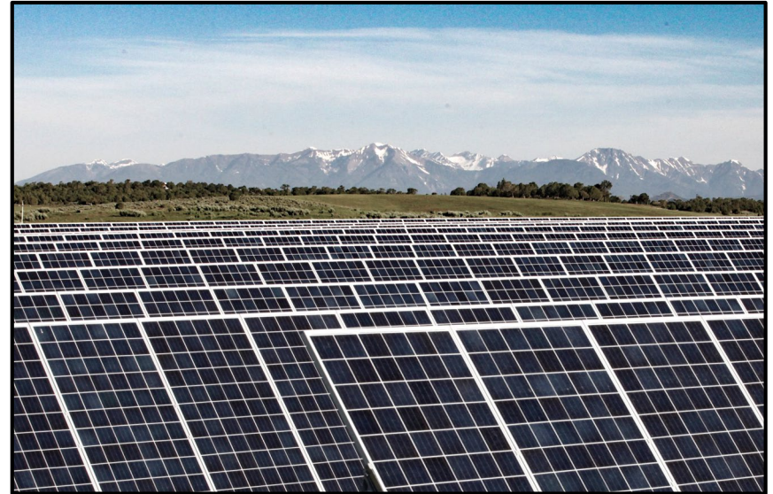
Southern Ute Indian Tribe (CO) Construction completed on the 1.3 MW Oxford Solar Project (June 2017).
