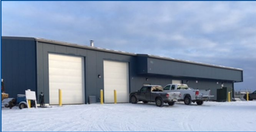
Council Of Athabascan Tribal Governments and Gwitchyaa Zhee Corporation (AK) Combined Heat and Powerhouse (below) and the Old Power Plant (top) (December 2017)
