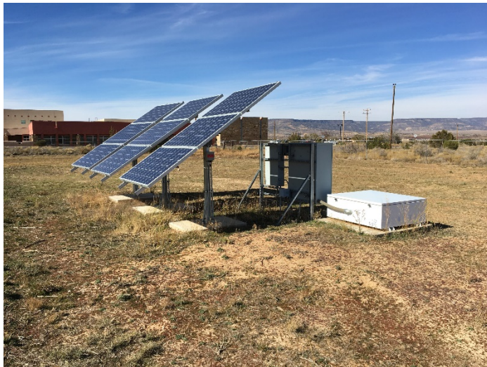
Off-grid pv system for running track lighting
