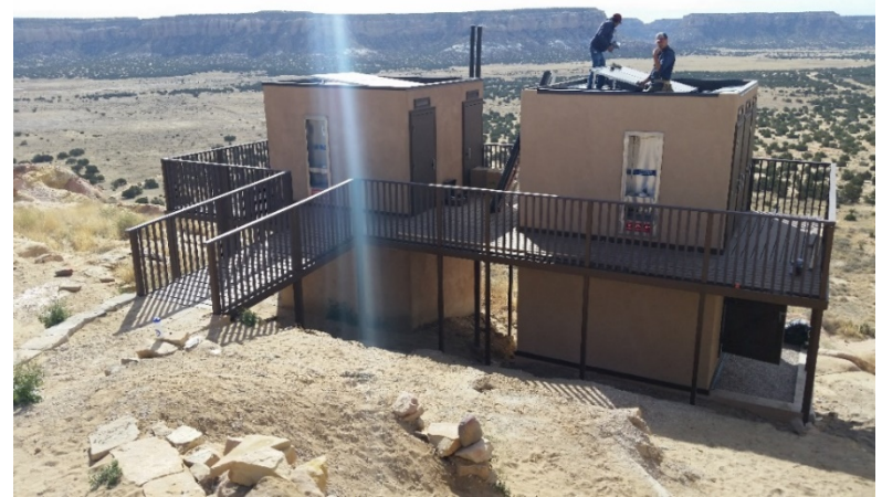
13 unit off-grid waterless composting restroom buildings atop Old Acoma
