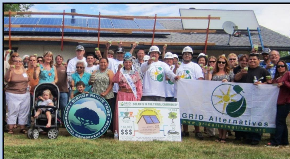
Photo: 1st rooftop solar installation – 2013
