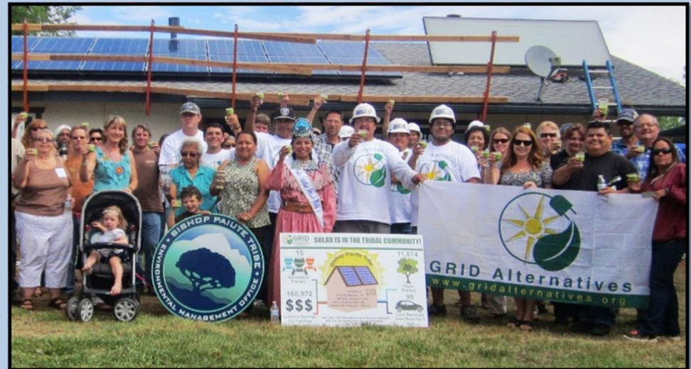
Photo: 1st rooftop solar installation – 2013
