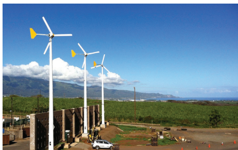
Photo courtesy of Cliff Ryden, Blue Pacific Energy, LLC
