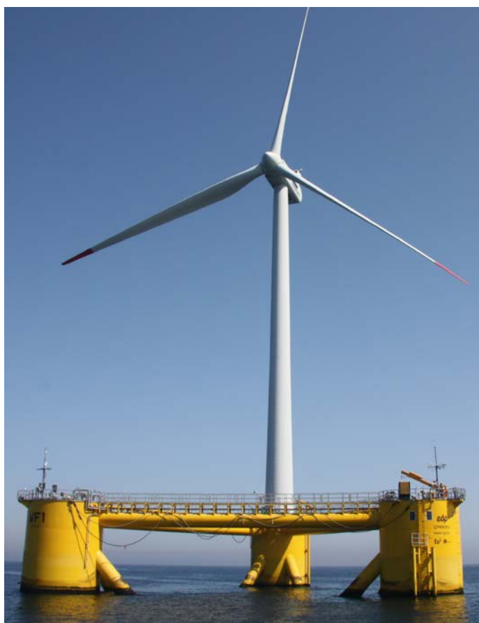
Shown here, WindFloat by Principle Power, Inc., is one example of the platform systems developed from oil and gas technology currently available to offshore floating wind project developers. The objective of the SpiderFLOAT system is to make it possible to tap more than 1,200 MW of U.S. deepwater wind resources more effectively than is possible with existing technologies. Photo by NREL
