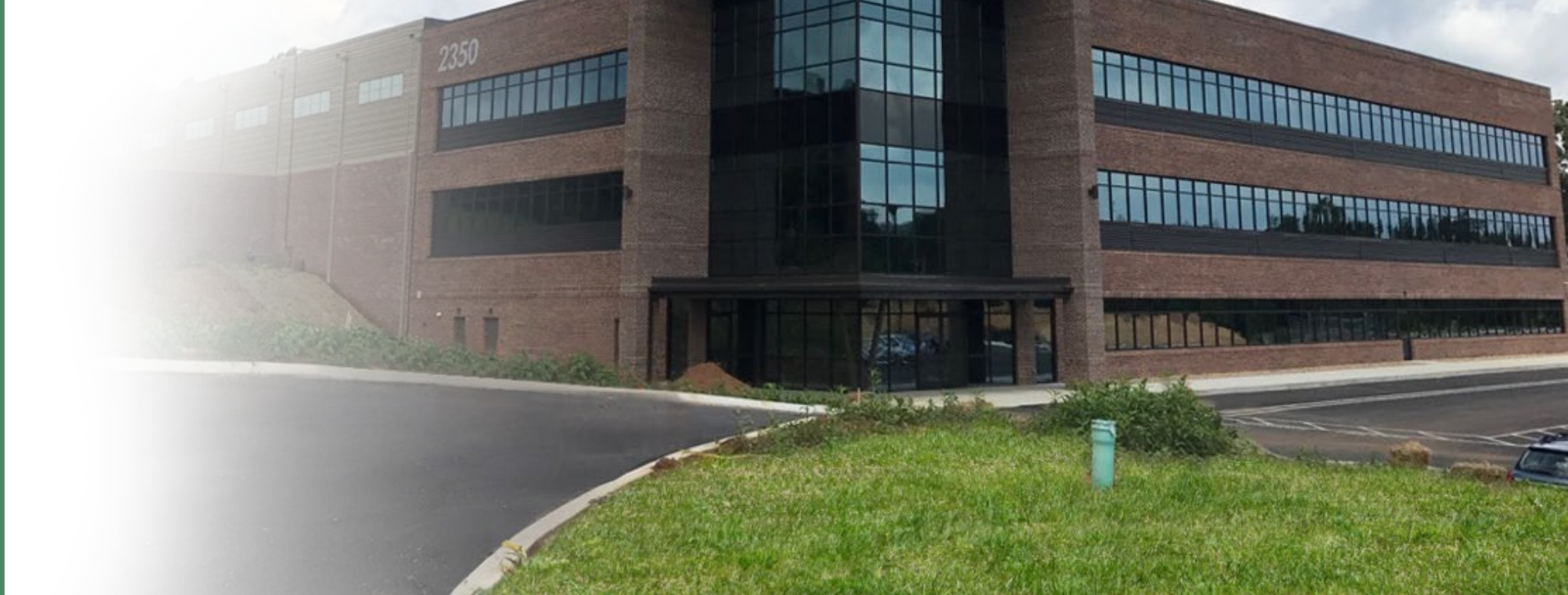
New facility 110,000 sq. feet total with 40,000 sq. feet of high bay
