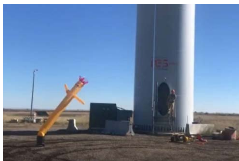
Deterrent at base of turbine
