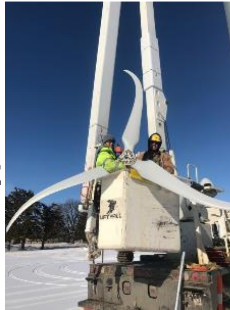
Turbine repair crew. Photo from South Dakota WAC
