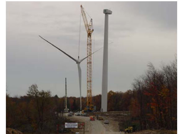
Construction of a wind turbines (Photo by Cris Hein)
