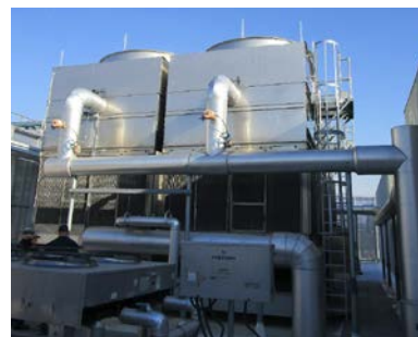
Example of a cooling tower
