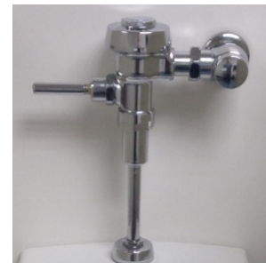
Diaphragm flush valve
