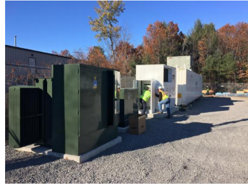
Workers install battery energy storage system in Sterling, MA.
