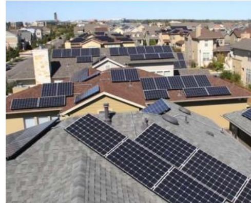
Residential PV portion of the Austin Energy distributed energy resource system.
