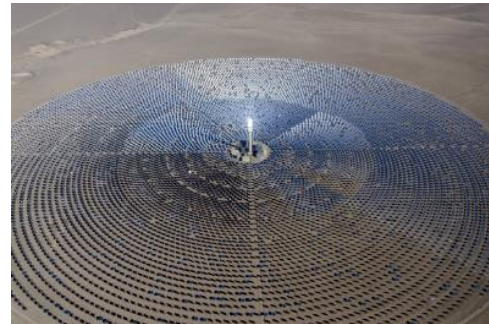
Crescent Dunes concentrating solar power plant with central tower heated by reflected light
