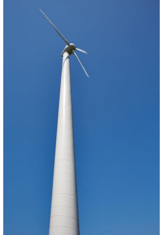
Installed first spiral welded tower
