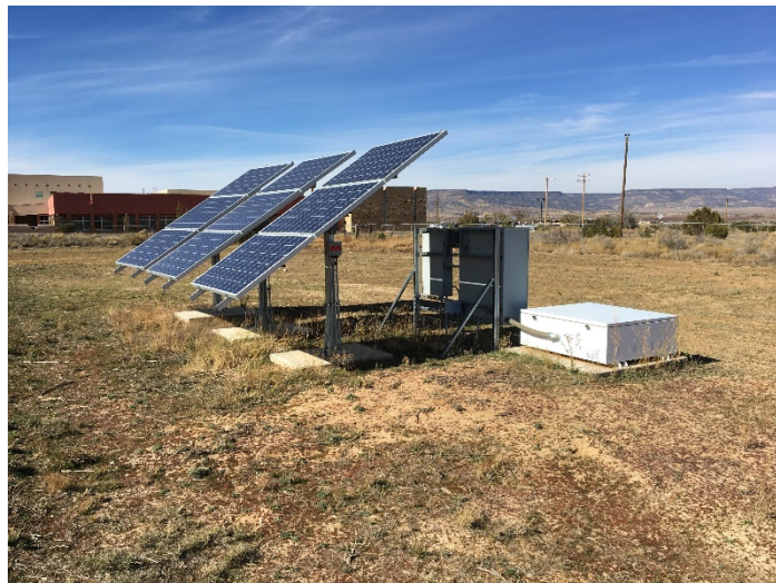
Off-grid pv system for running track lighting
