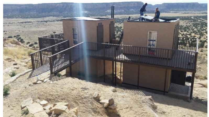
13 unit off-grid waterless composting restroom buildings atop Old Acoma
