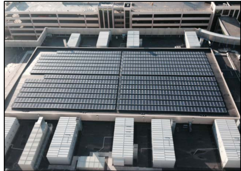
Forest County Potawatomi Community (WI) 922.95 kW community solar project. A 447.64 kW installed on the Potawatomi Bingo Casino in Milwaukee (shown right) and 22 kW installed in the Tribe's Land and Natural Resource building in Crandon (shown above)
