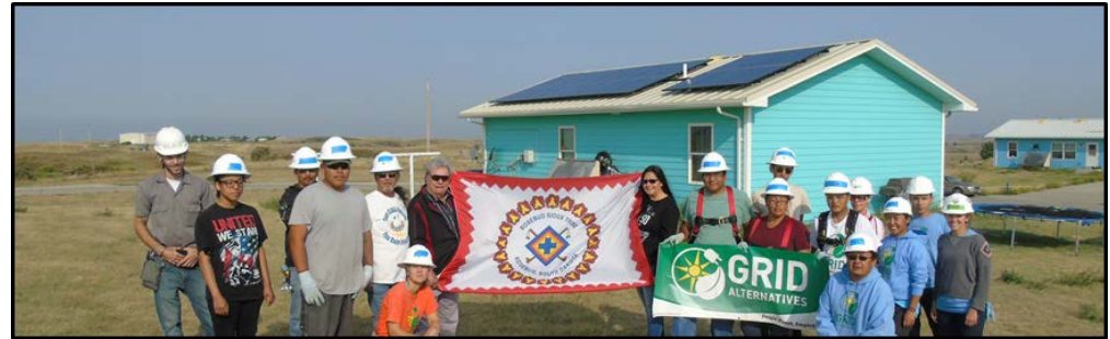
Rosebud Sioux Tribe (SD) installed a low-income residential system (August 2016)
