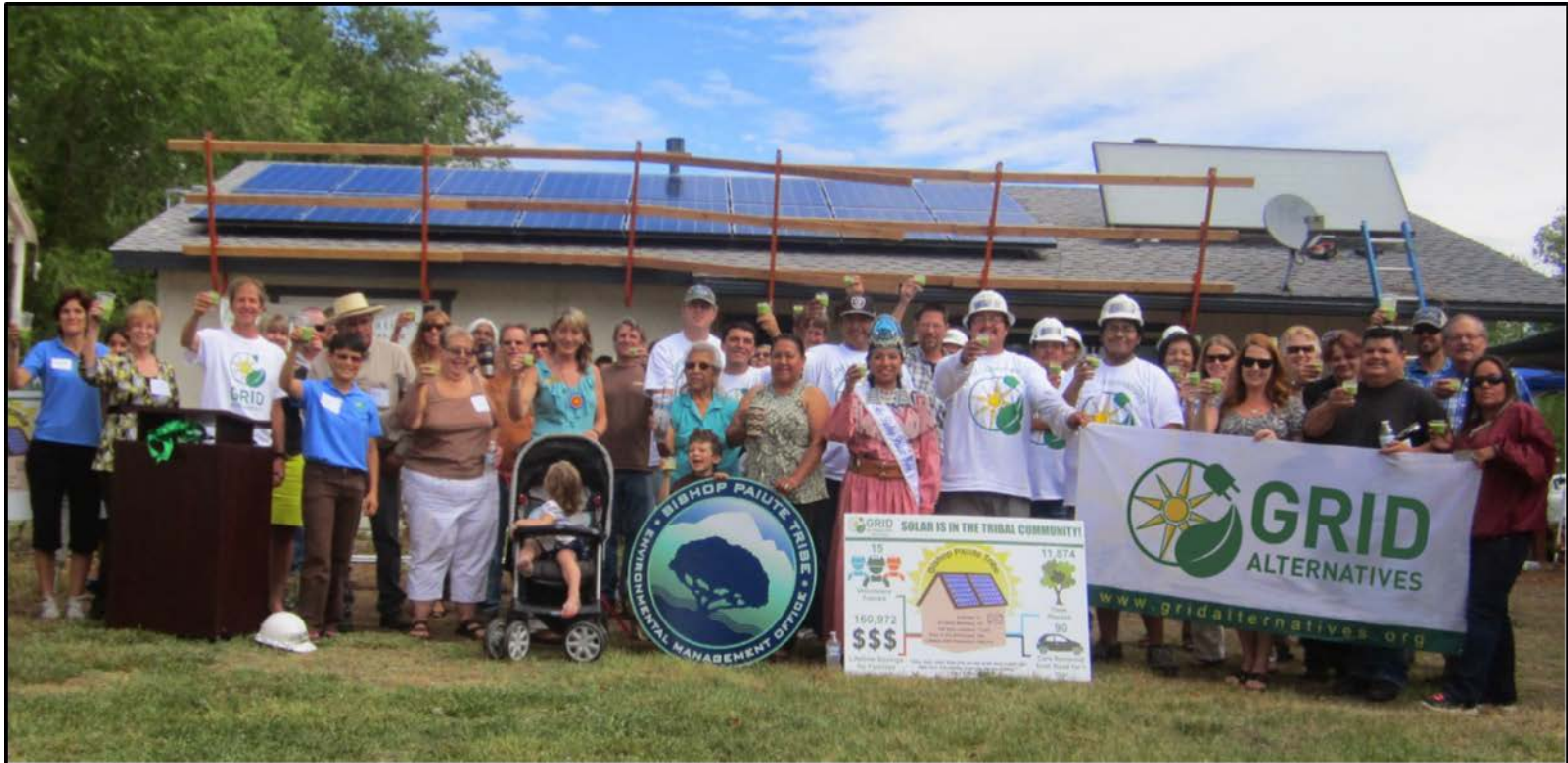
The Bishop Paiute Tribe (CA) Residential Solar Program with two grants from DOE will install 178 kW on 56 homes (2015)
