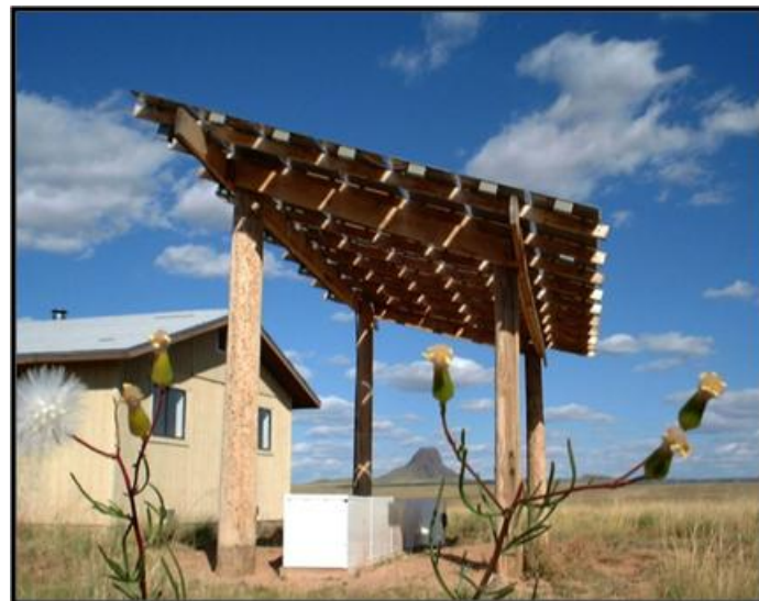
Solar arrays on home on the Navajo Nation
