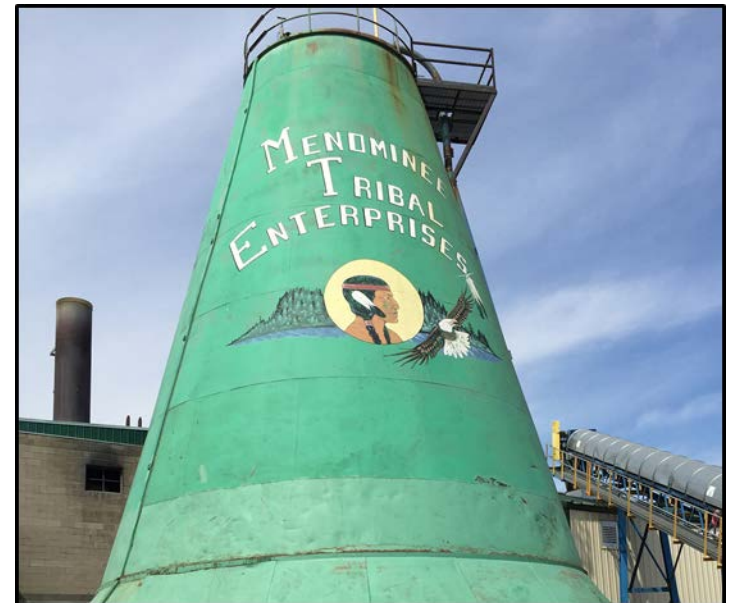
Menominee Tribal Enterprise (WI) Biomass CHP (April 2016)
