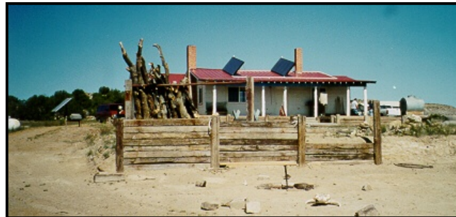
Solar Installations at Pueblo of Laguna's Majors Ranch (NM)
