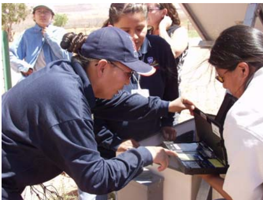
Figure 2: Picture of Field Visit to NTUA with Vircynthia Charley. Vircynthia takes readings from a PV installation using her laptop. Pictured from left to right: Vircynthia Charley, Melissa Parrish, and Deborah Tewa.
