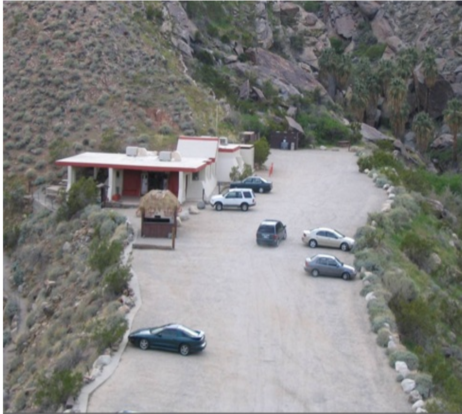
Photo showing Trading Post prior to PV installation, taken from Eastern view. Source: Mineral Assessment Program Phase II
