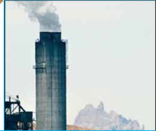
Four Corners Power Plant
