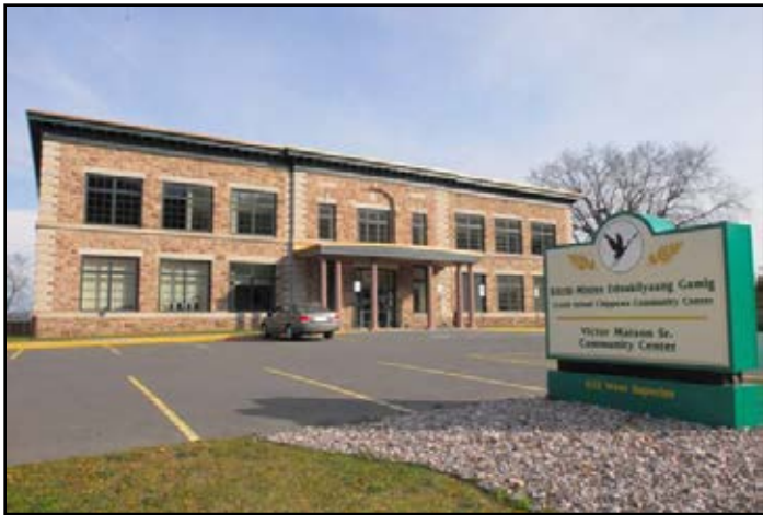
Sault Ste Marie's Tribal Health Clinic and Community Center, one of 45 buildings which will have energy audits (MI)
