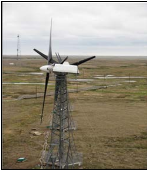
Chaninik Wind Group's Thermal Heating Project (AK)
