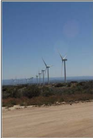
Campo Band's Wind Farm DOE funding Phase II (160 MW)
