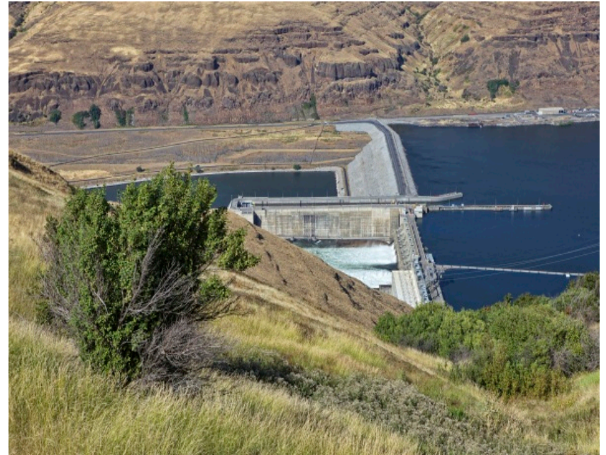
Lower Granite Dam
