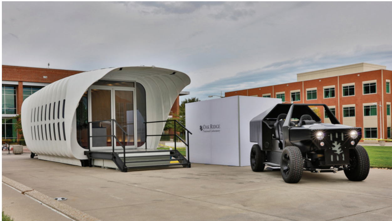
Figure 6.A.8 The Additive Manufacturing Integrated Energy (AMIE) Demonstration project at ORNL is exploring the potential for AM to expand the design opportunities for improved energy utilization between the buildings and transport sectors. 55
