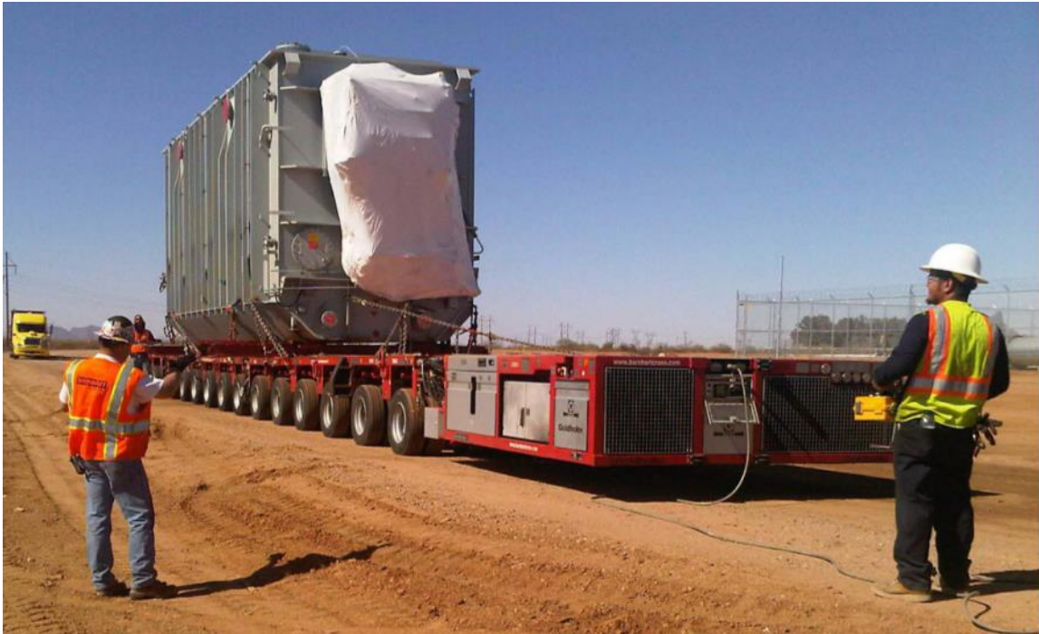
LPT delivery via road by Barnhart
