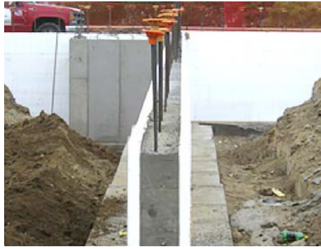
ICF wall construction
