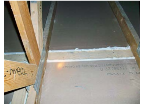
Air-sealed top plates before attic insulation
