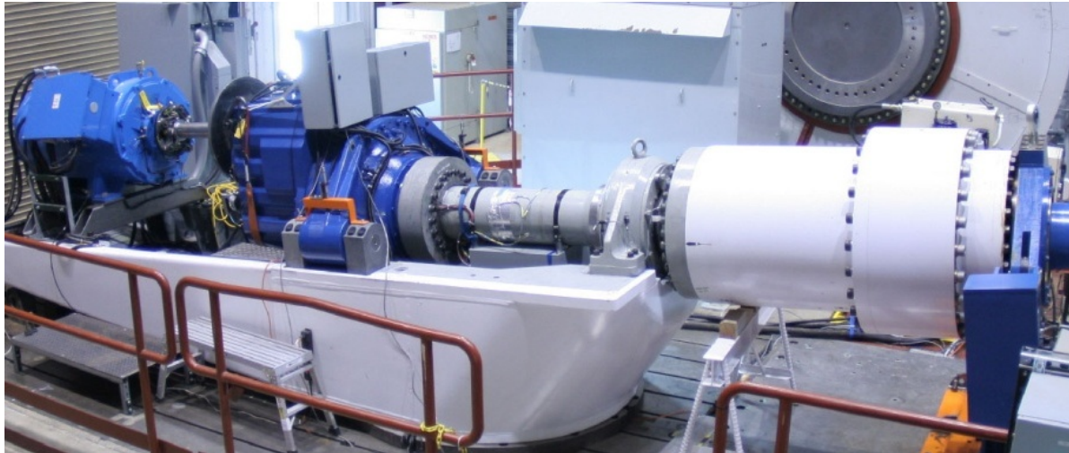
GRC Drivetrain with existing gearbox in NWTCC 2.5 MW Dynamometer
