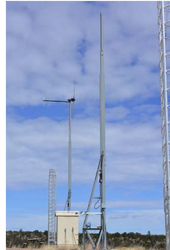
Coupled Wind Turbines
