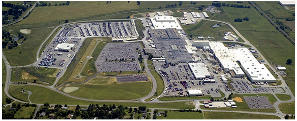
Volvo Trucks New River Valley Plant in Dublin, Virginia.
