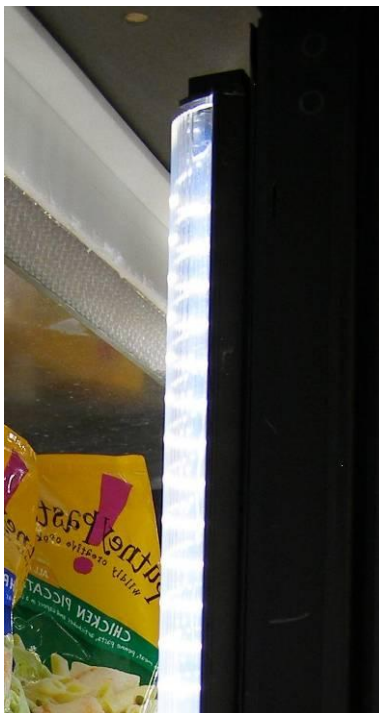
Figure 1. Top of LED Power LED strip as installed
