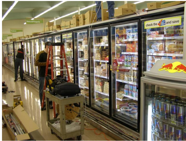
Figure 3. LED strip installation starting at one end of row
