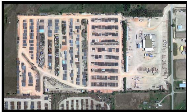
Figure 22: Typical Construction Staging and Equipment Areas (Photo courtesy of Robert M. Donnan, http://www.marcellus-shale.us/ )
