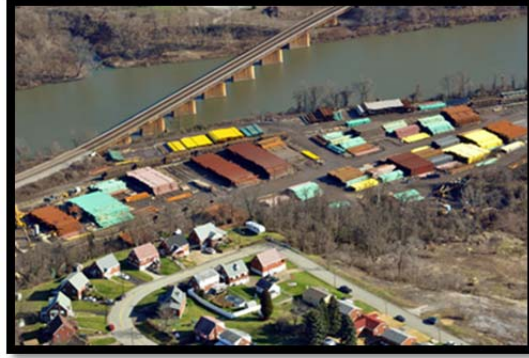
Figure 23: Pipe Storage Facility in Pennsylvania (Photo courtesy of Robert M. Donnan, http://www.marcellus-shale.us/ )
