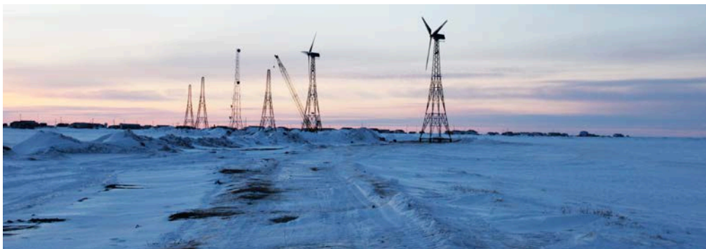
Wind turbines installed in Kwigillingok, Alaska, as part of the Chaninik Wind Group Multi-Village Wind Heat Smart Grid Project. Photo from Intelligent Energy Systems, NREL 29204
