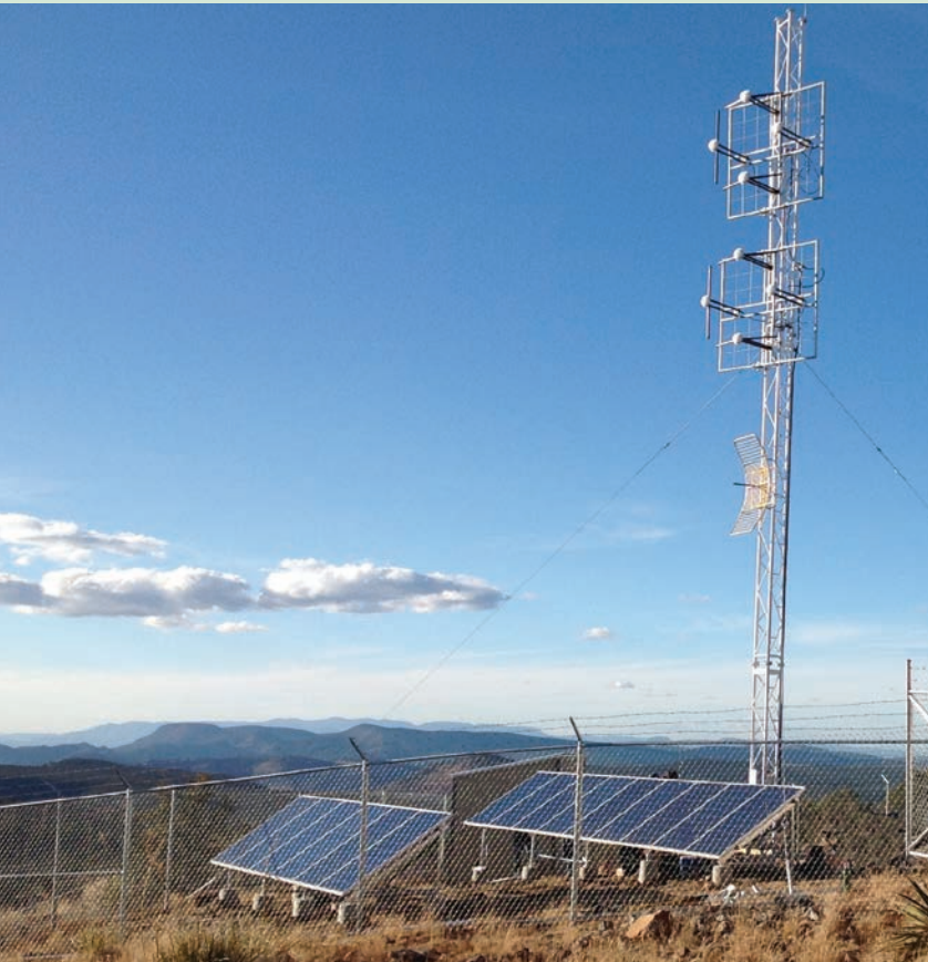
The San Carlos Apache Tribe is making use of its extensive solar resources to power tribal facilities, including this 10-kilowatt (kW) solar PV system, which generates energy to run the tribal radio tower. Photo from San Carlos Apache Tribe, NREL 29202
