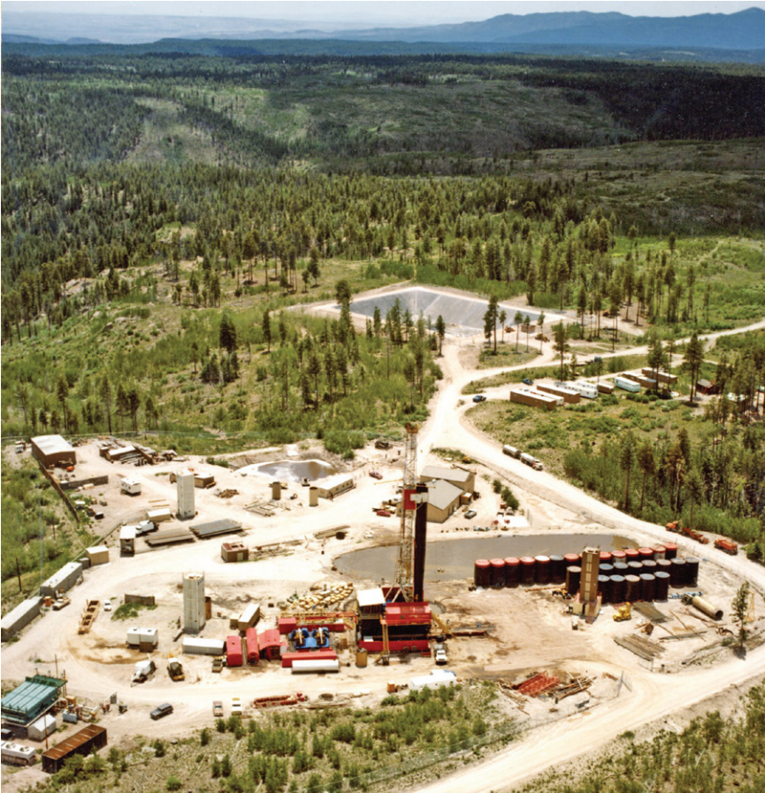
Figure 10. Fenton Hill, New Mexico Hot Dry Rock program site
