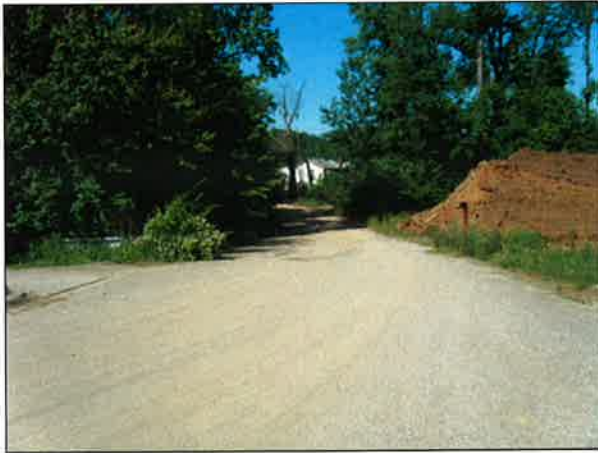
View of construction entrance (southeast) from Formex Rd facing west.
