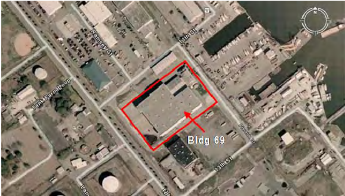
Figure 2-3: Location of Building 69 within the Charleston Naval Complex
