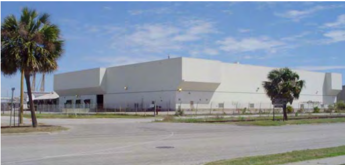
Figure 2-4: Street View of Building 69 Source: Kelly et al, 2009.
