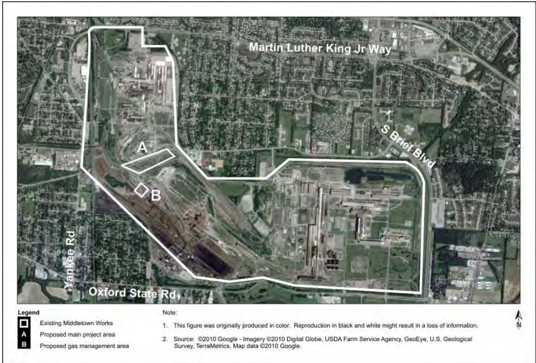
Figure 2-2. Satellite view of the Middletown Works and vicinity showing the site boundary and location of the proposed project.
