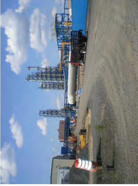
Photograph 5. Northern view of adjacent Phase I polysilicon production facility
