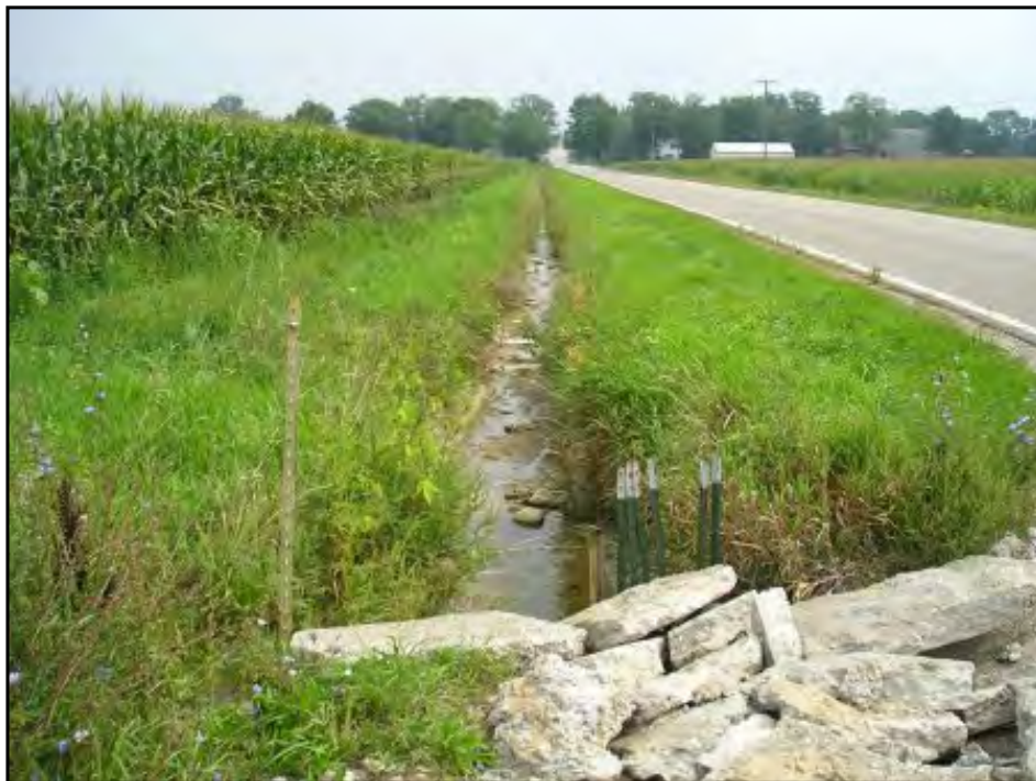
VIEW OF DRAINAGE DITCH/SWALE LOCATED ALONG SOUTHERN PROPERTY BOUNDARY, FACING EAST
