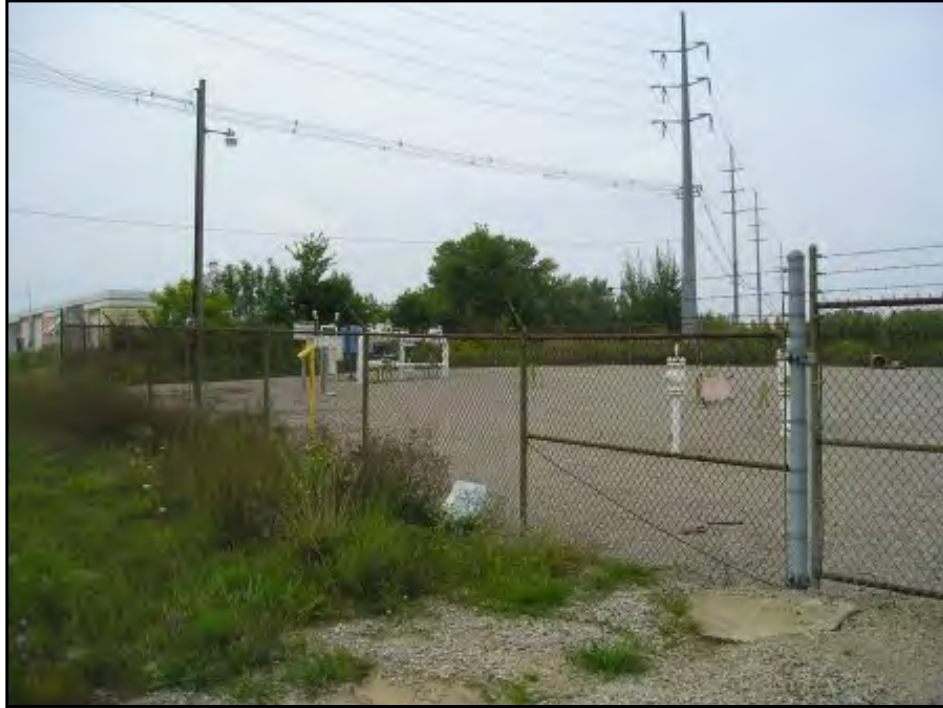
VIEW OF SEMCO GAS PIPELINE, POWERLINES, AND RAILROAD LOCATED ADJACENT TO THE SOUTHWEST AND WEST OF THE SUBJECT SITE, FACING NORTHWEST
